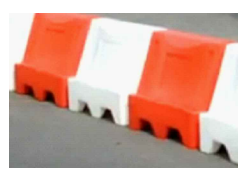
Typical temporary barrier
